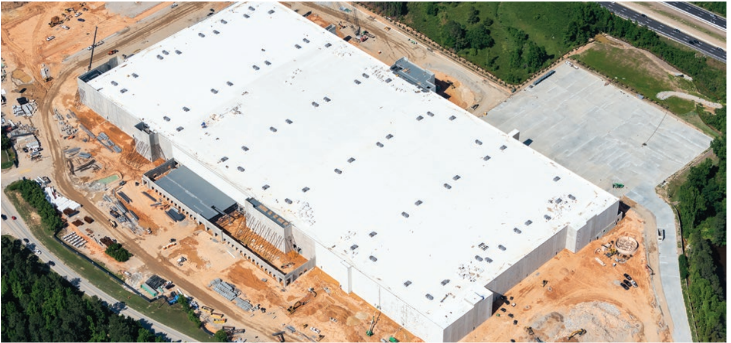
Amazon facility being constructed on the Garner Technology Center site
