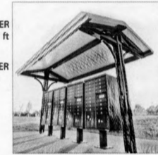
MAIL KIOSK EXAMPLE THE CANOPY PROVIDES AT LEAST 4' OF COVERED AREA BEYOND THE FRONT PLANE OF THE MAIL BOXES
