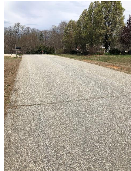
Transverse Cracking.
