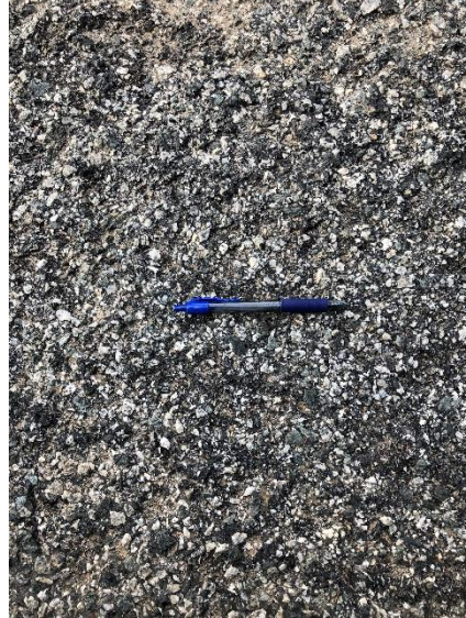
High Severity Raveling
