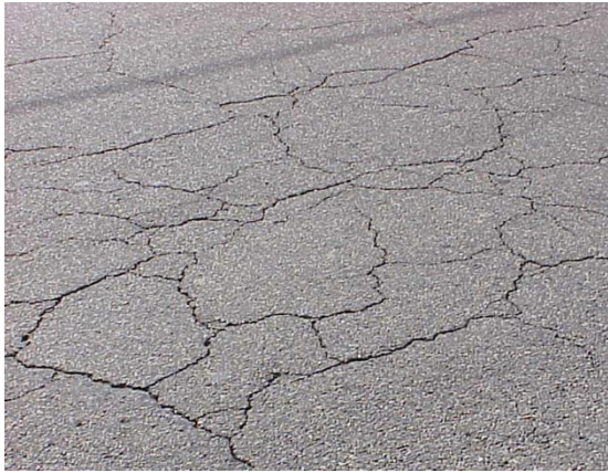
Medium Severity Block Cracking
