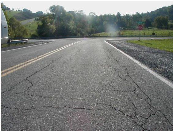
Medium Severity Fatigue Cracking.
