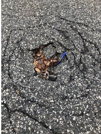
High Severity Pothole
