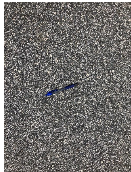
Low Severity Raveling
