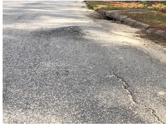
Medium Severity Roughness
