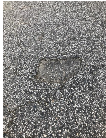
Medium Severity Pothole
