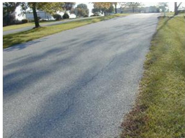
Low Severity Fatigue Cracking.
