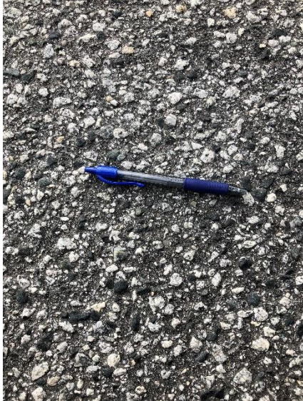
Medium Severity Raveling
