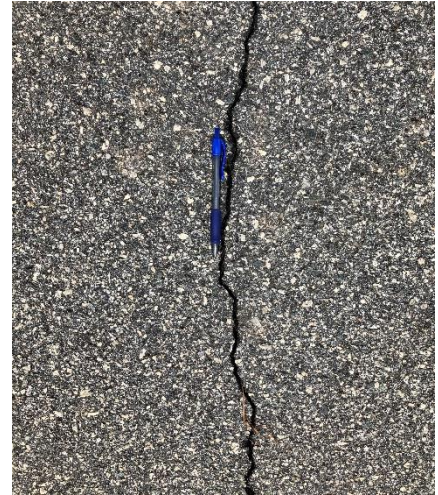
Low Severity Transverse Cracking.
