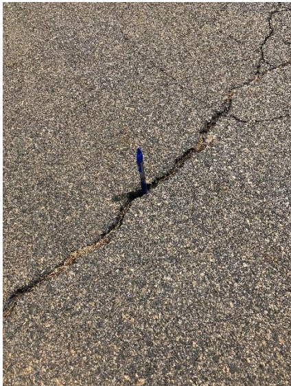
Medium Severity Transverse Cracking.
