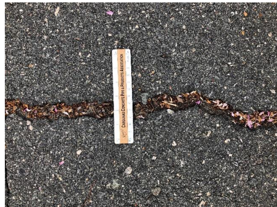
High Severity Transverse Cracking.
