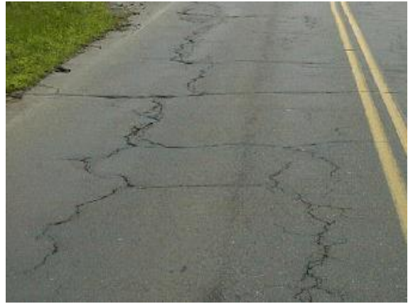
High Severity Block Cracking
