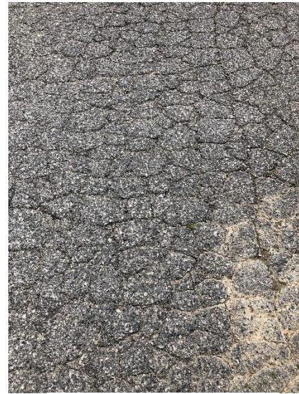
High Severity Fatigue Cracking.
